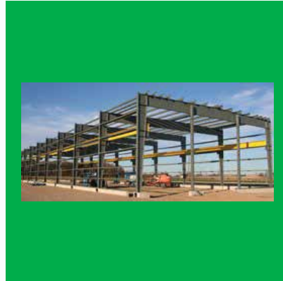
Pre Engineered Building
