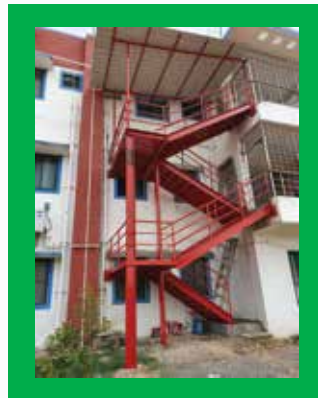
Emergency Exit Grill Staircase
